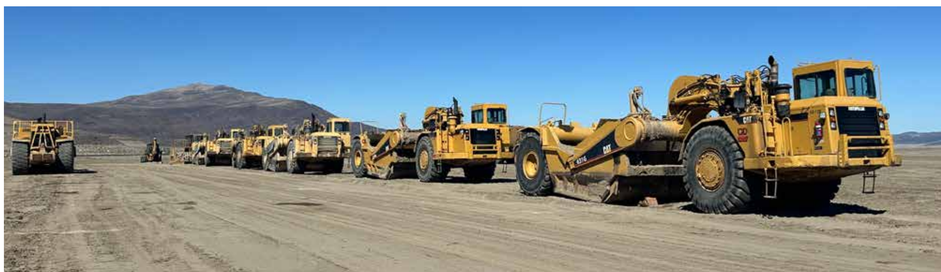
Scrapers line up at the Victory Logistics District site as crews continue grading work for Mark IV Capital's rail spur project. Photo by Robert Perea
