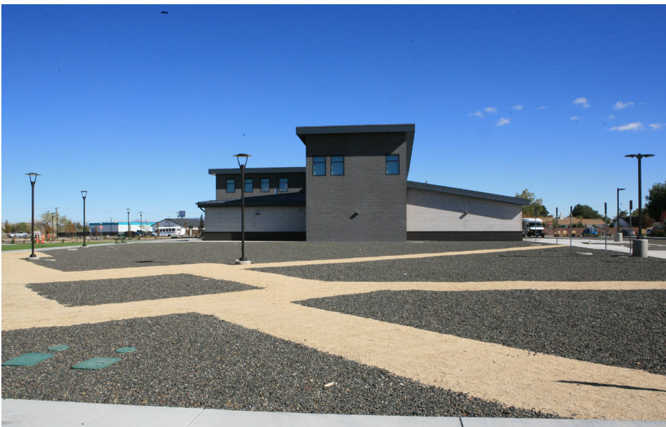
The Fernley City County approved the ground lease for the site of the Early Learning Center, shown here with the Community Response and Resource Center in the background. Photo by Kerry Lyman
