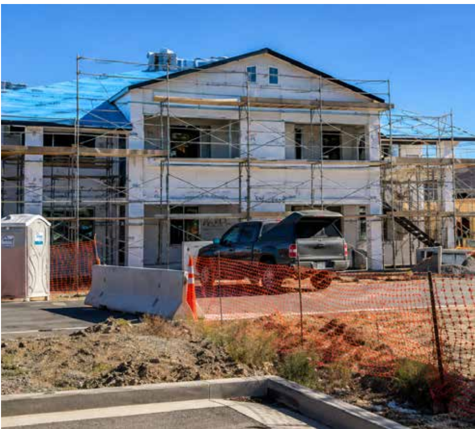
Construction abounds throughout Fernley as projects get underway. Photo courtesy of City of Fernley.
