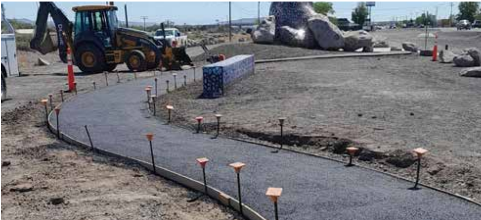
The Fernley City Council voted to wait until getting final costs for the building of the Community Response and Resource Center before allocating money to complete the Main Street Art Park. Photo courtesy of the City of Fernley
