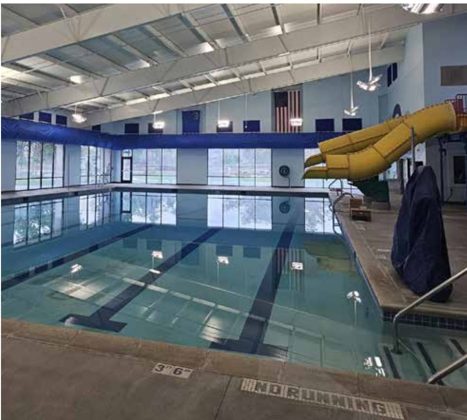
The Fernley pool opening has been delayed due to an electrical failure. Photo courtesy of Desert Surge Swim Club.
